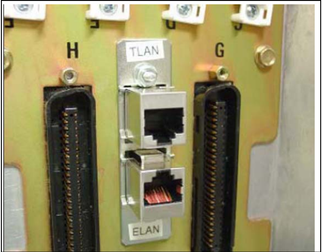
Figure 41 Installed Ethernet port adapter plate
